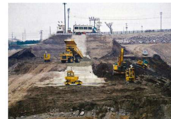
Photo 5 RCC method by unmanned construction
