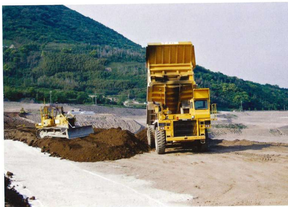
Photo 10 Delivery of sediment and spreading (1 layer: 50 cm)
