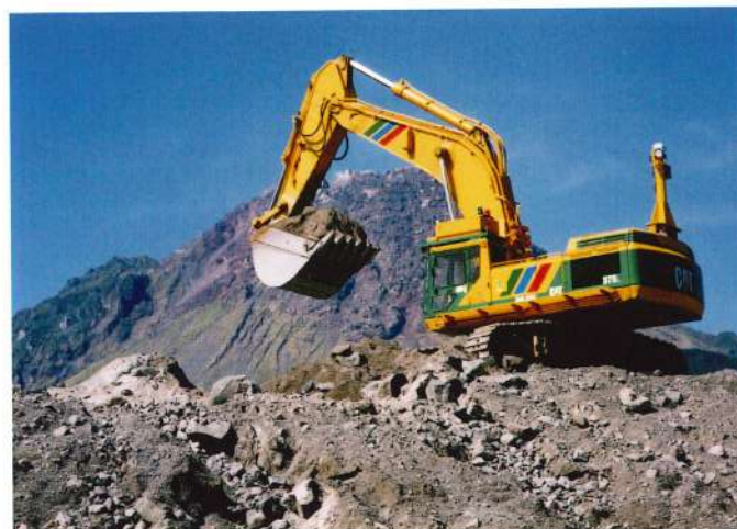
Photo 4 Removal of sediment by unmanned construction technique
