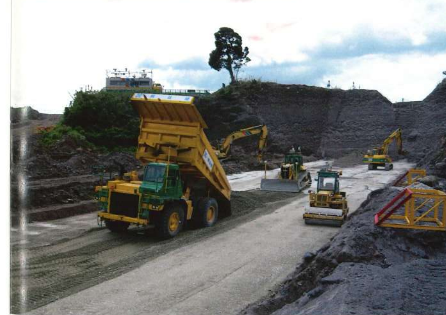
Fig. 22 New technology for the sabo works. "the unmanned construction method"
