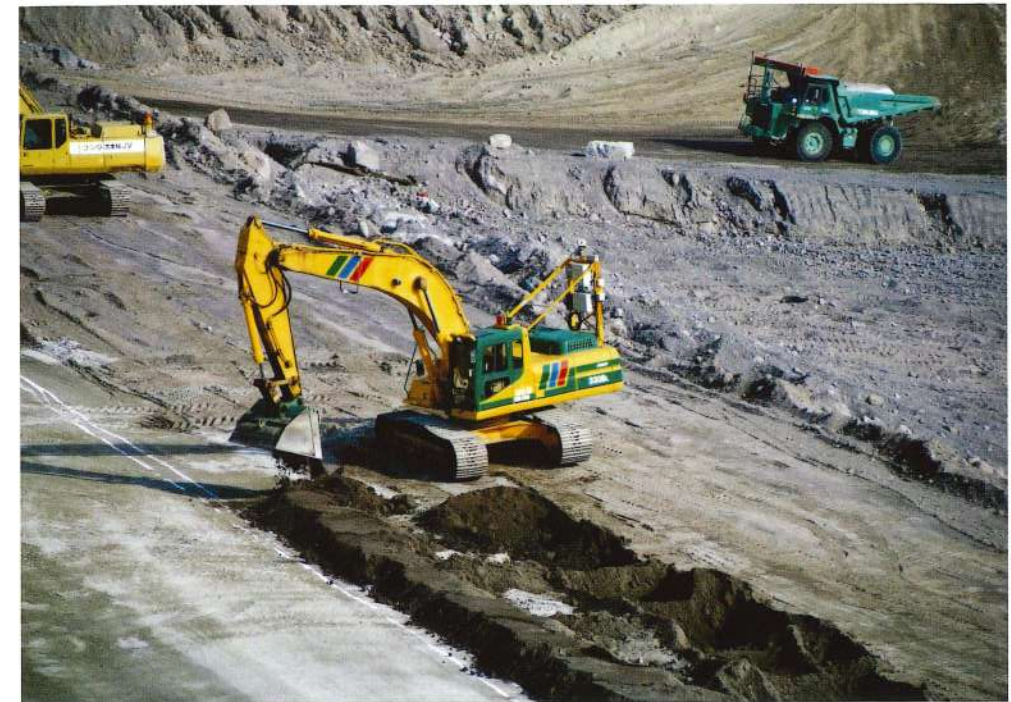
Photo 11 Shaping of sediment for use as forms
