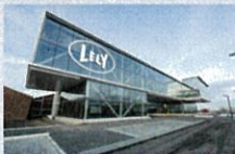
Lely Group, Maassluis Optimal control with Priva ecoBuilding
