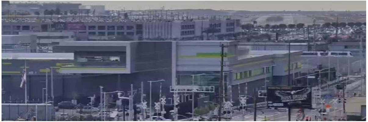
Consolidated Rent-A-Car Facility (ConRAC)
