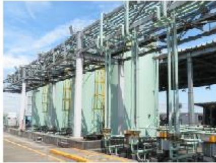
Waste oil emulsion fuel production facility
