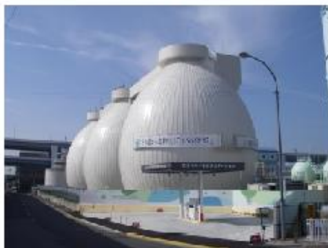
Biogas station attached to a sewage sludge digestion facility
