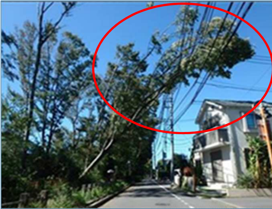
Fallen trees leaning on power lines, causing power outages
