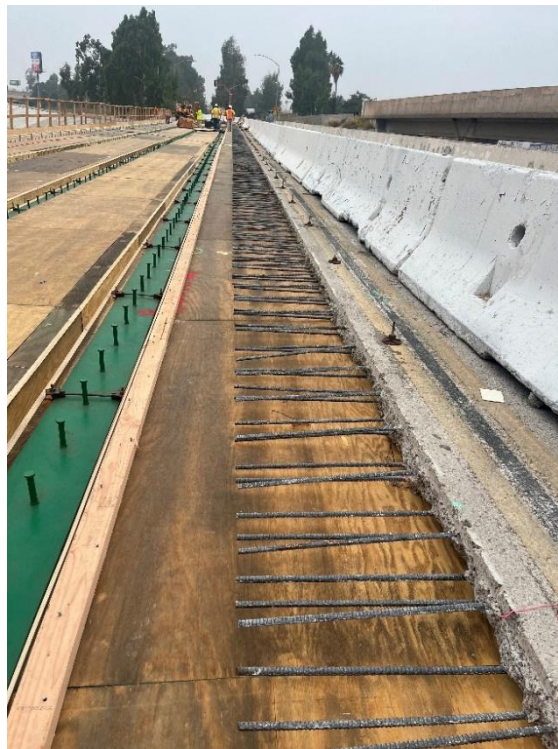
既有橋面板鋼筋及鋼梁剪力釘保留完好(Rio Houdo Busway Bridge )
