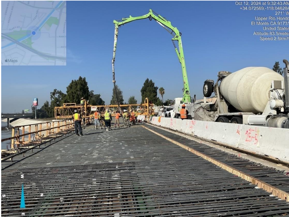
輕質混凝土澆置 (Rio Houdo Busway Bridge )
