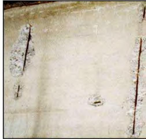
Coatings, Inhibitors and Cathodic Protection may be Applied to Foundations with Less Damage
