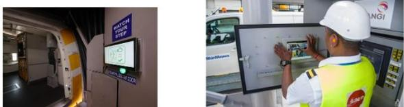
A new remote control panel on the ground allows a single operator to complete the full docking process
