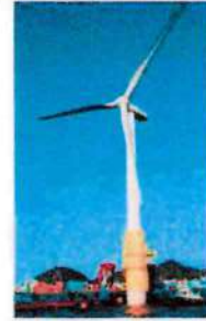
Wind turbine: 2MW Downwind type (Operation started 2013)
