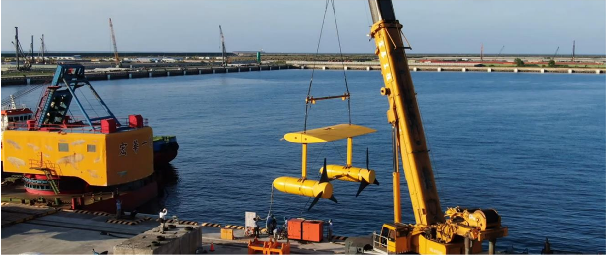
Launching of the Generator Using Lifting Cranes.
