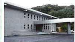
[Maintaining positive pressure in a facility] [Enhancing performance of emergency power generators] [Installing switchboards for power supply vehicles] [Renewing other facilities]
