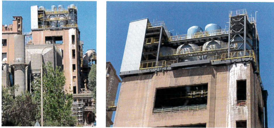
Figure 16. Overview of preheater building (left) and completed superstructure (right).
