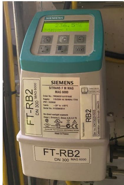
貨油泵輸出流量計SENSOR (041502H503)
