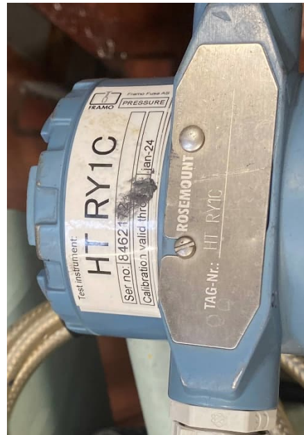
Pump Head Sensor(8462172)
