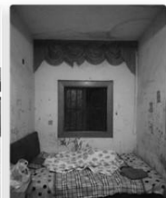
Mess caused by the former tenant
