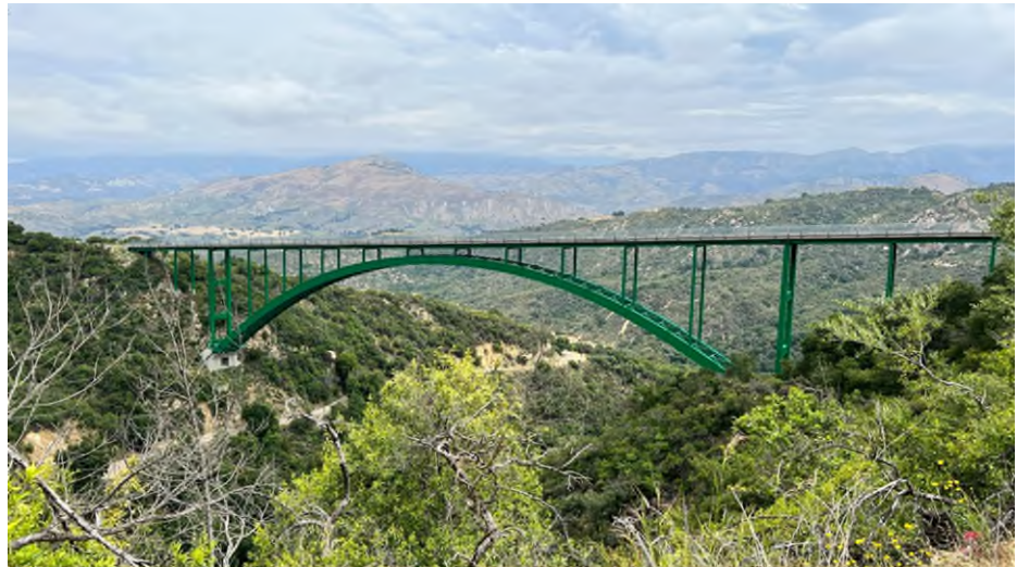
圖 58 Cold Spring Canyon Arch Bridge
