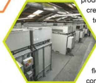
Located adjacent to the hydrogen production plant, EMEC's energy storage building houses 48 vanadium flow battery (VFB) modules with a combined storage capacity of 1.8 MWh.
