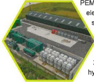
Based on the electrolyser running at full power for 24 hours, up to 260 kg of high purity, fuel cell grade hydrogen can be generated.
