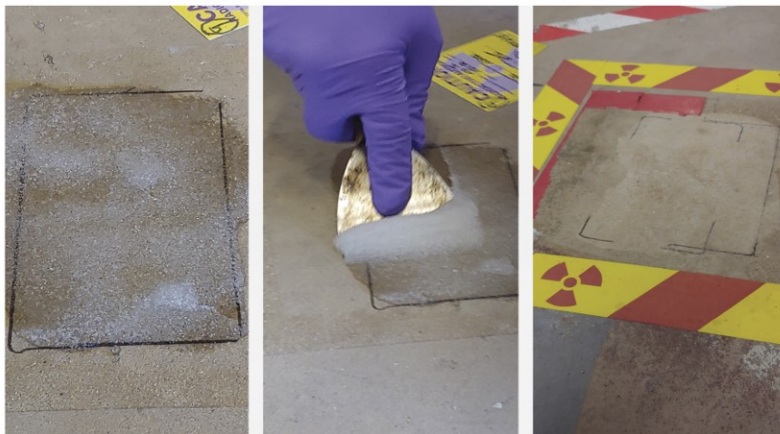
圖 17 自乾式高分子凝膠示範操作圖(Source: Ofra Paz Tal, Decontamination Processes and Techniques: Polymeric Gels)
