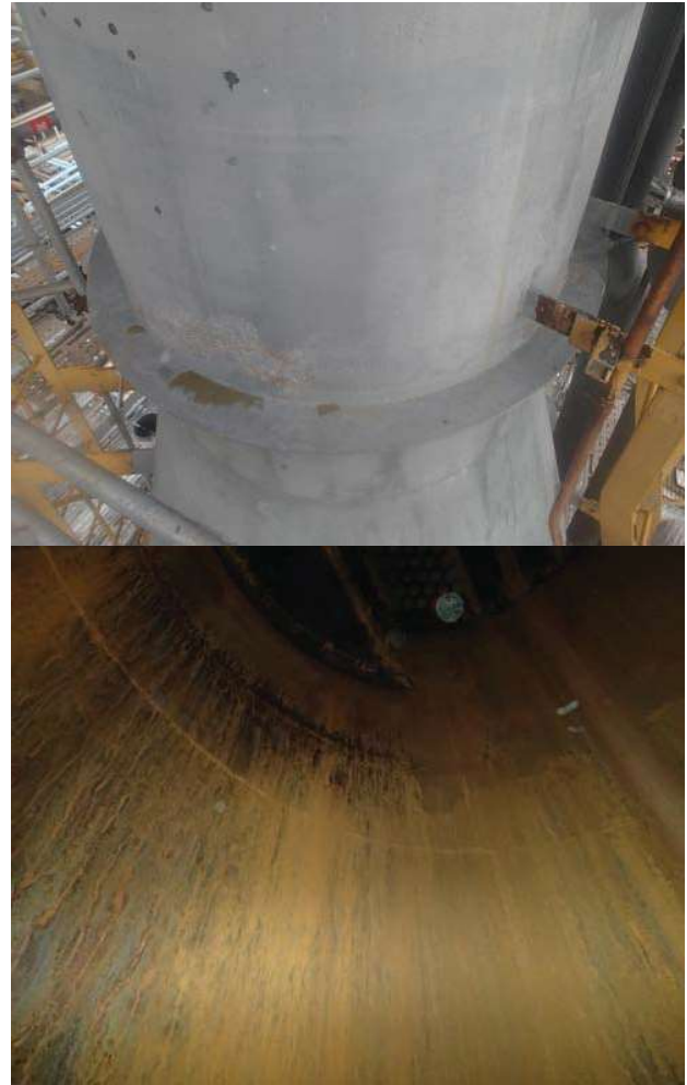
Figure 10: External and Internal Appearance @ DA-3202 S1
