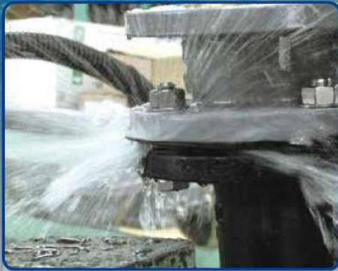
The problem comes from loosening nuts caused by earthquake vibration or by uneven pressure distribution from inconsistently tightened bolts.
