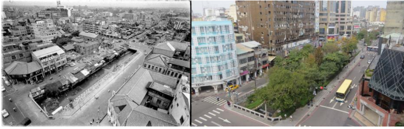
Figure 7. Comparison of the Luchuan Irrigation Canal with the WEI-Luchuan (1971 left vs 2021 right). (Yu Ru-ji and TIIWE)
