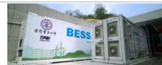
Fig.3 The 2M/1MWh short duration application EESS II
