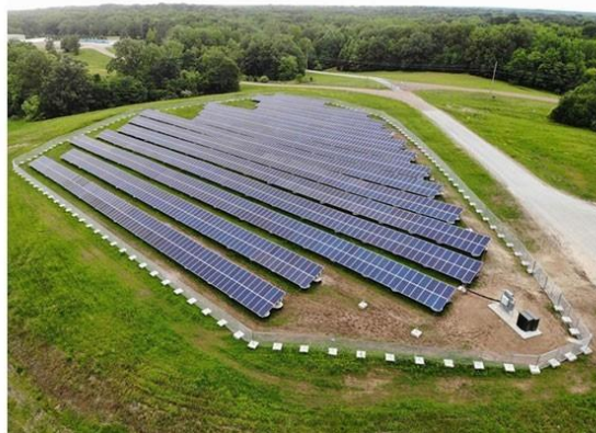
A 2.7-MW solar farm constructed on a portion of a landfill in Somerville, Tennessee, USA (Source: https://www.wastetodaymagazine.com/article/tennessee-landfill-solar-project-complete/ )
