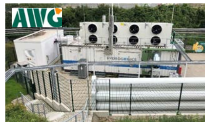
AWG Wuppertal (DE) – 400,000 tpy 1 MW Electrolysis (100 m 3 /h H 2 )
