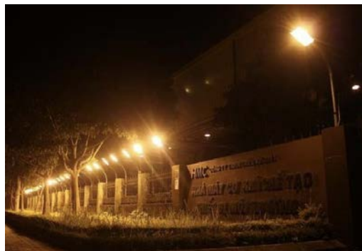
Lighting system at the Dong Van I Industrial Park run by Syngas-powered internal combustion engine generator from waste gasification for 7 consecutive days
