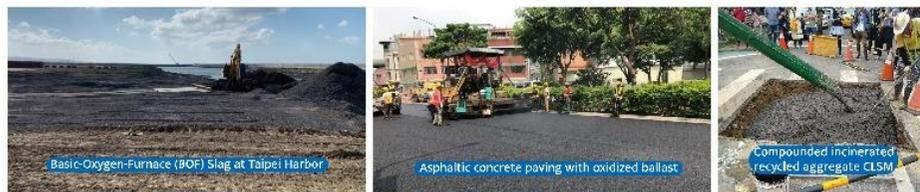
Inorganic recycled resources can be recycled in construction engineering, related projects include ready-mixed concrete aggregates, asphalt concrete aggregates, controlled low-strength materials (CLSM), cement products, brick raw materials (red bricks, tiles), paving works base-level aggregates materials, land reclamation materials, cement substitute raw materials, etc.
