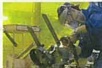
08 Construction Steel Work
