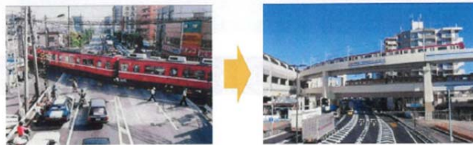
Removed the level crossing at Daiichi Kaihin
