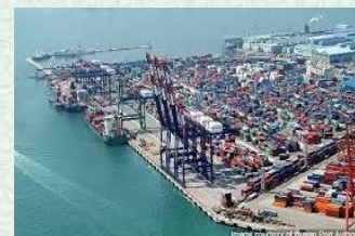
Construction of Seaport, River Port and Dry Port
