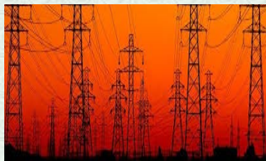
Power Generation, Transmission and Distribution
