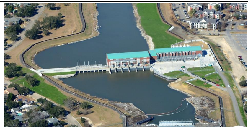
London Avenue PCCP
