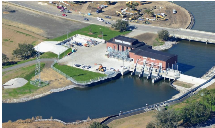
Orleans Avenue PCCP
