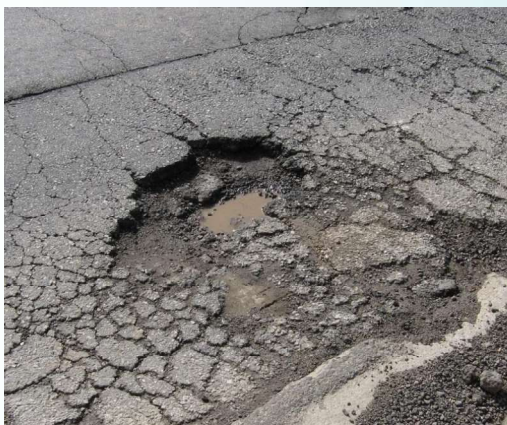
Severe pothole and good patching (Photo taken by DGH)
