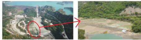
▲ Fig 3 Temporarily pool contains dredging mud. It contained 40K m 3 of mud each round. 3 round each year, resulted maximum 120K m 3 every year.
