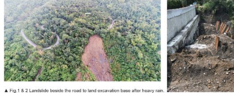
▲ Fig 1 & 2 Landslide beside the road to land excavation base after heavy rain.
