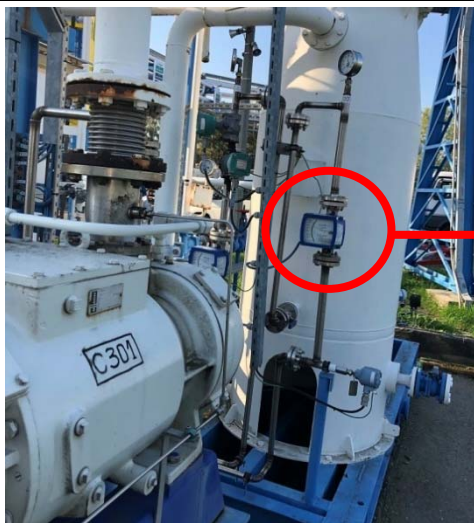
圖 10. Coolant Flow Meters (for vacuum pump and vapor temperature management)
