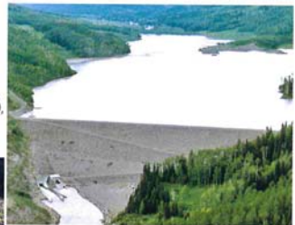
Ridgeway Dam - Ridgeway Dam of the Dallas Creek Project, a rolled-earthfill dam was constructed on the Uncompahgre River in 1987.
