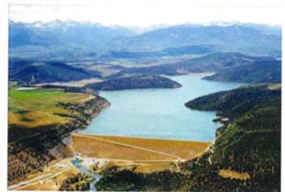
Ridgeway Dam - Ridgeway Dam of the Dallas Creek Project, a rolled-earthfill dam was constructed on the Uncompahgre River in 1987.
