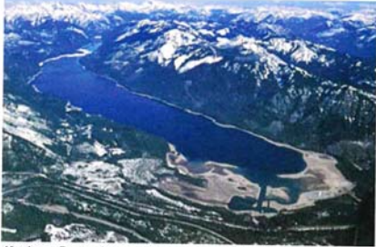
Kachess Dam - Construction was completed in 1912. It is a zoned earthfill dam with a height of 115 feet (35 meters) with a crest length of 1,400 feet (426.7 meters). Seepage issues are being monitored. Simulated dam safety exam will be conducted.
