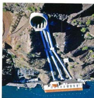
Havasu Pumping Plant, Parker, Arizona.
