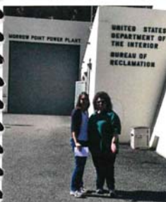
Morrow Point Dam - 12 miles downstream from Blue Mesa Dam, Reclamation's first thin-arch, double-curvature dam.
