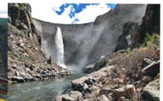
Morrow Point Dam, 12 miles downstream from Blue Mesa Dam, is Reclamation's first thin-arch, double-curvature dam.
