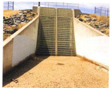
Reach 11 Dikes, located near Phoenix, Arizona.
