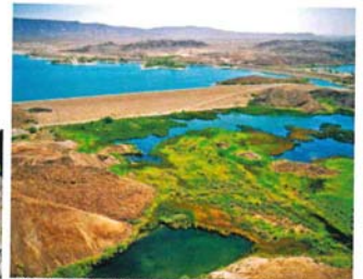
Senator Wash Dam, located about 18 miles northeast of Yuma, Arizona, on the California side of the Colorado River.
