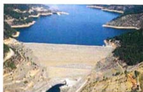
Trinity Dam - located on the eastern Klamath plate, the oldest and easternmost of four eastward-dipping thrust sheets that comprise the Klamath Mountains province.
