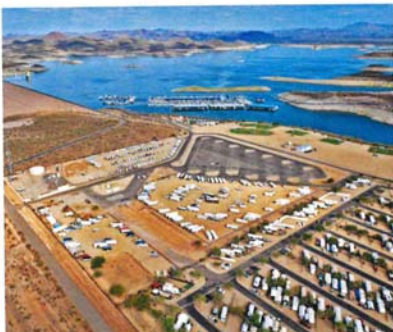
New Waddell Dam, Phoenix, Arizona.
