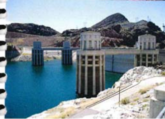
Hoover Dam - Hoover Dam and Lake Mead, spanning the Arizona-Nevada state line, are located in the Black Canyon of the Colorado River about 56 kilometers (35 miles) southeast of Las Vegas, Nevada. It is a concrete thick-arch structure, 221 meters high (726.4 feet) and 379 meters long (1,244 feet).
