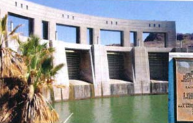
Parker Dam - a concrete arch dam with a structural height of 97 meters. Only 28 meters of the dam's structure is visible since 73 percent of the dam's structural height is below the original riverbed.
