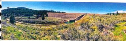
Boca Dam - completed in 1939 and has a height of 116 feet and a crest length of 1,630 feet. It provides flood protection for Reno and Sparks, Nevada.
