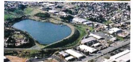
Martinez Dam - Constructed in 1947, it is an earthfill dam with a structural height of 62 feet (19 meters) and a crest length of 1,200 ft. (366 meters).
