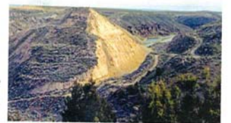
Teton Dam, a 100-m-high embankment dam, completed in November 1975, failed catastrophically on June 5, 1976.
