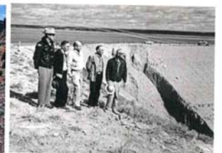
Fontenelle Dam, suffered a near failure due to seepage erosion in September, 1965.
