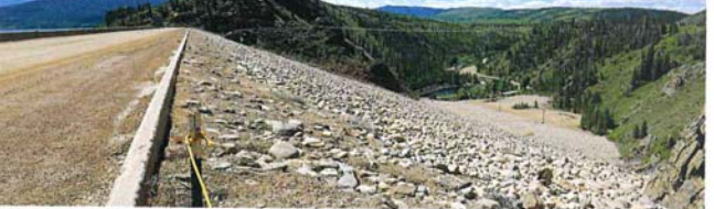
Granby Dam - Granby Dam is located on the Colorado River about 9.6 kilometers (6 miles) northeast of Granby, Colorado. It collects and stores most of the project water supply, including the flow of the Colorado River and water pumped from Willow Creek. There are 3,877 meters (12,722 feet) of auxiliary dikes. The reservoir has a capacity of 666 million cubic meters (539,800 acre-feet).
