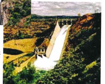
Echo Dam - Construction completed in 1931. It is a zoned earthfill dam with a height of 158 feet (48 meters) with a crest length of 1,887 feet (575 meters). A powerplant was installed in 1987. The primary purpose of the dam is water conservation, however, it is also used for recreation purposes. Water from the Echo reservoir is released into the Weber River and is diverted into 41 privately built canals and laterals leading to the irrigable land.
