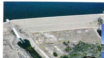
Starvation Dam is a zoned earthfill dam located three miles northwest of Duchesne, Utah on the Strawberry River.
