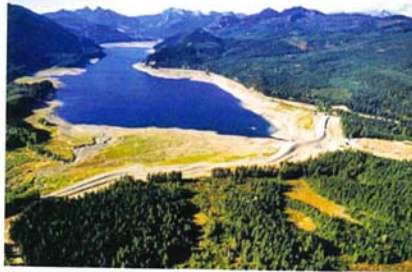
Keechelus Dam - Construction was completed on 1917. It is a zoned earthfill dam with a height of 128 feet (39 meters) with a crest length of 6,550 feet (1,996.4 meters). Modifications are planned to address internal erosion caused by seepage.
