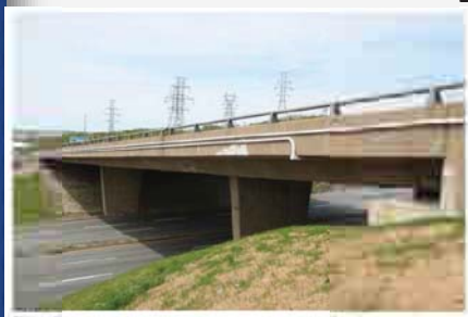
Figure D30: Victoria Road Overpass (VRO) – General View
