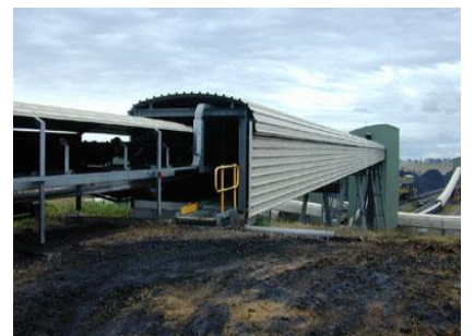
Entering crushing station
