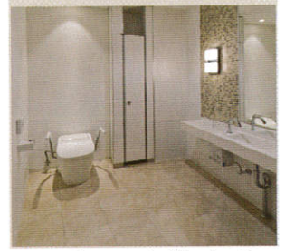
Water- and power-saving fully automatic self-cleaning toilets are installed.
