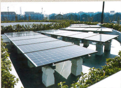
Rooftop solar panels provide electric power in emergencies. They will be able to provide electricity for three days in emergencies.
