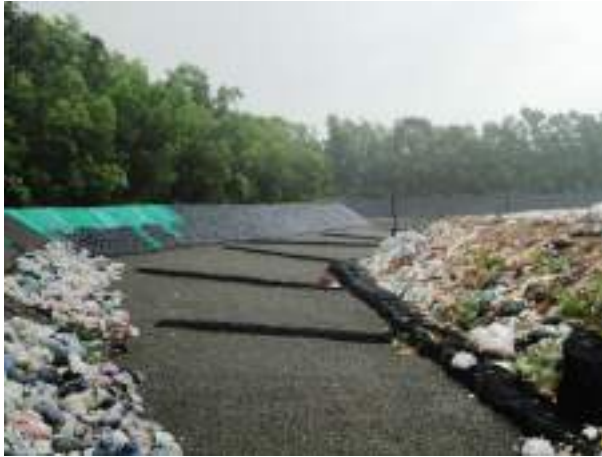
1 st Sanitary Landfill started in 2014 20 Metric Tons/ Day
