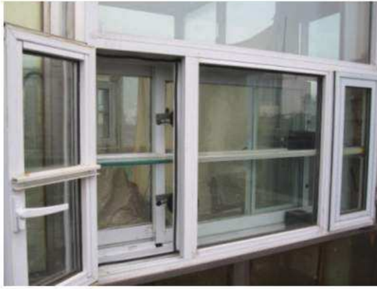
Natural ventilation ANC windows – plenum type
