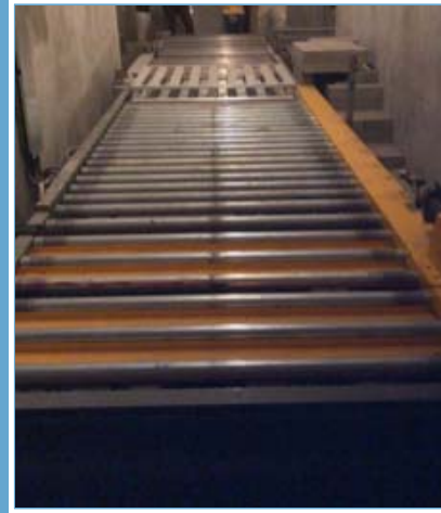
Pallet Conveyor With Slave Pallet In Maze Area Of Bunker
