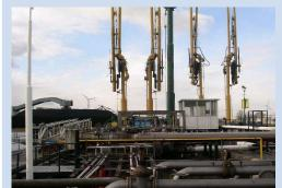
化學船卸載用機械設備(Liquid cargo equipment)
