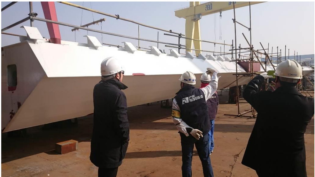
鋼橋外觀檢視
