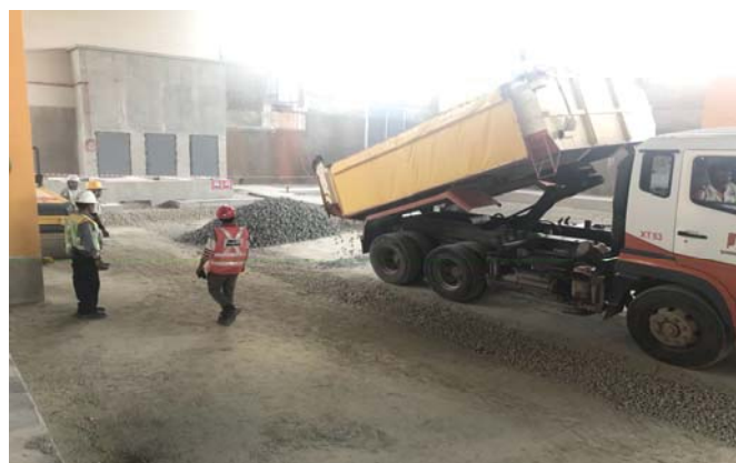
Ballast Laying in Zone 1
