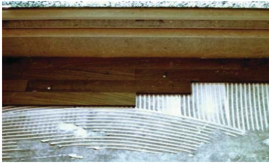
Timber Flooring Installation
