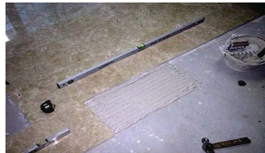
Stone / Tile Installation
