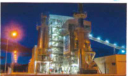
Biomasa de Cantabria at Reocin BFB boiler
