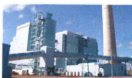
Basin Electric Dry Fork Station CFB scrubber
