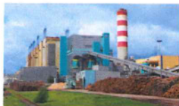
Polaniec Power Station CFB boiler
