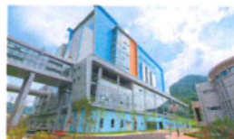
Green Energy Centre CFB boiler
