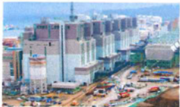
Samcheok Green Power Plant CFB boiler
