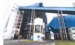
SINOPEC Projects CFB boilers
