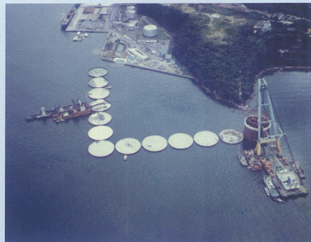
Construction of the reinforced shore using steel sheet pile cells
