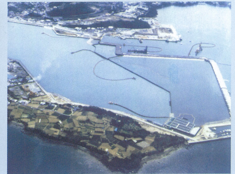
Dredging using a cutterless pump dredging ship
