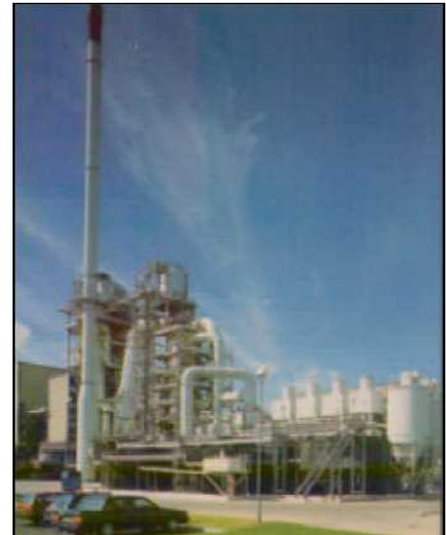
Waste Incineration Facility
