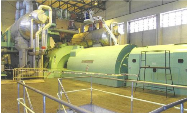
Initial status of the operations plant, Turbine Building
