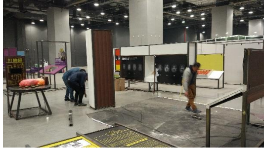
展品鐵件架構搭設完畢
