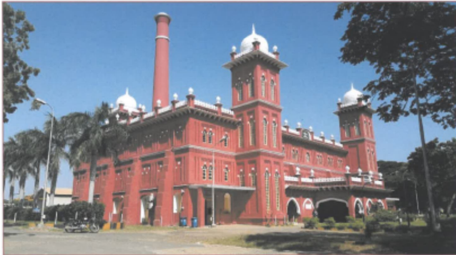
KILPAUK WATER TREATMENT PLANT
