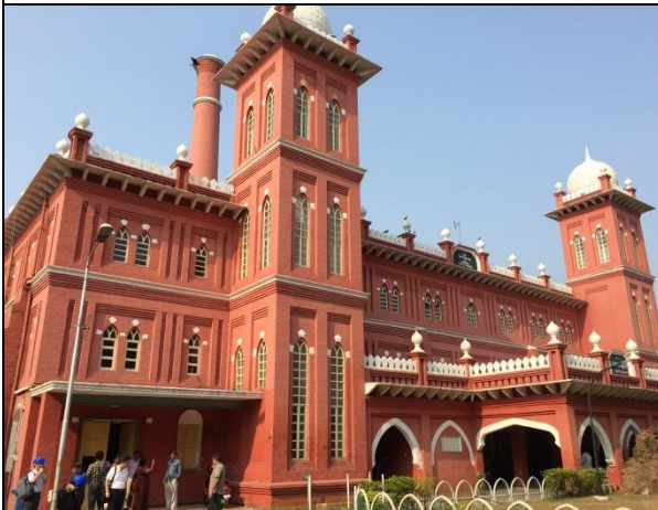
圖 43 Kilpauk water treatment plant
