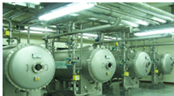
Cheng-Ching Lake WTP Ozoneation Facility
