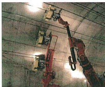
Situation of inspecting the internal condition of tunnel lining
