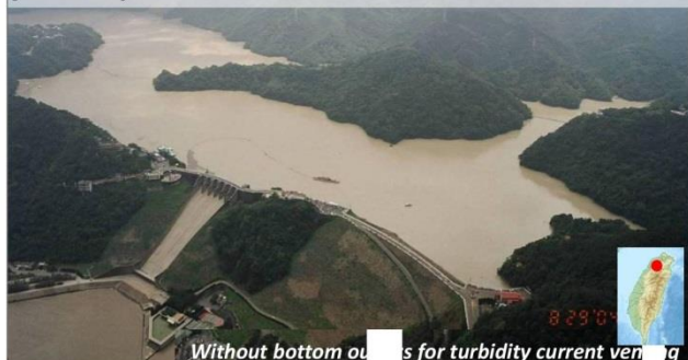
Without bottom outlets for turbidity current venting
