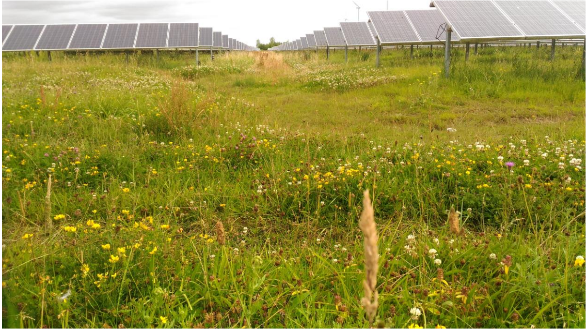
PHOTOGRAPH 3-4. 5MW Solar PV project of Case C.
