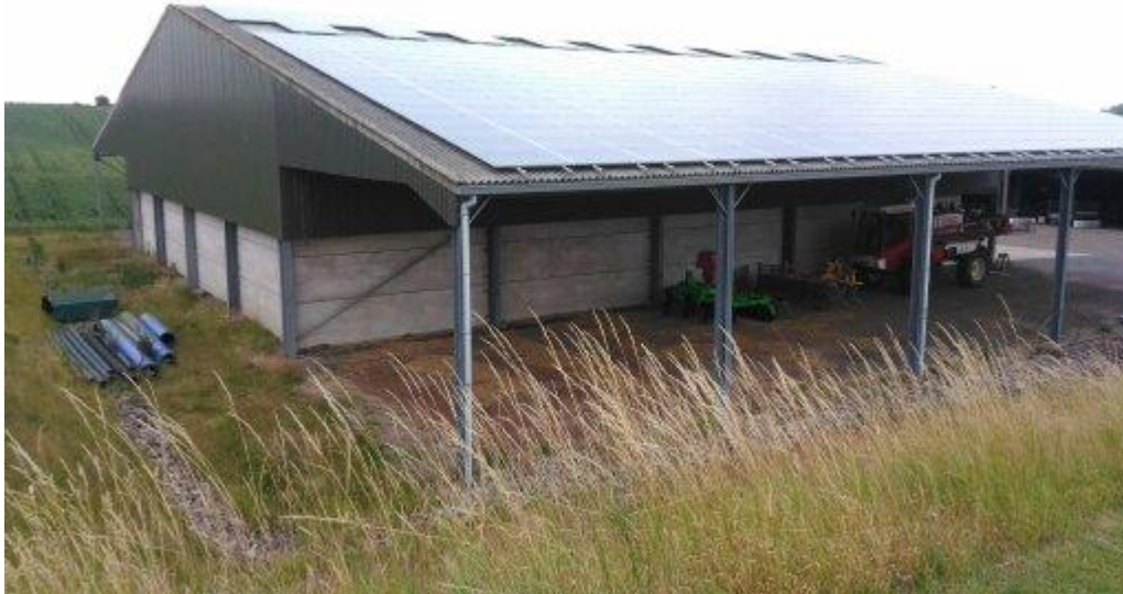
PHOTOGRAPH 4-5. Solar PV project of Case B is mounted on building roof, instead of farmland.
