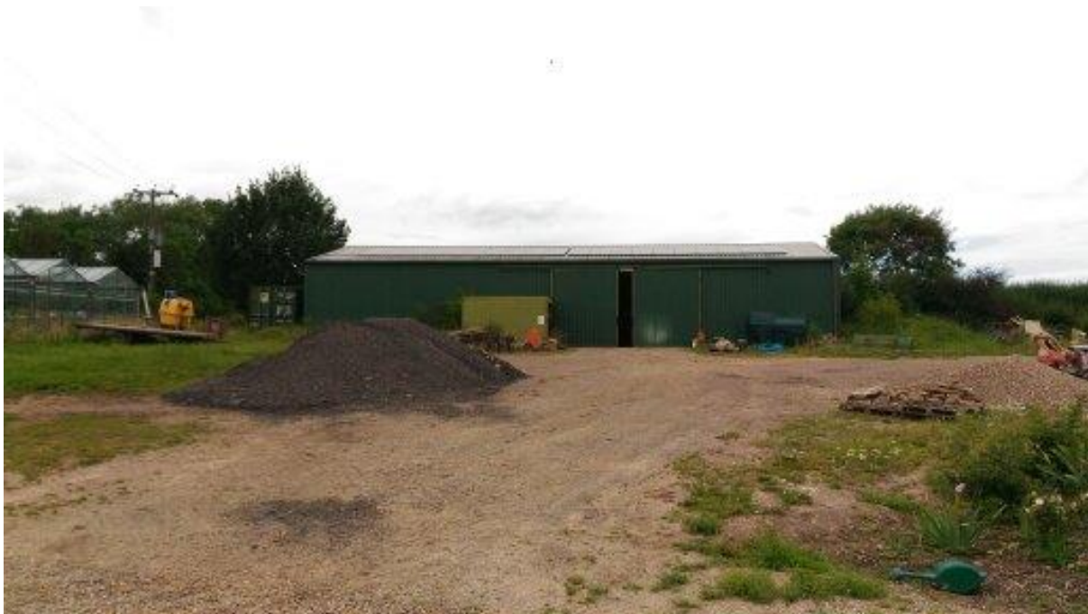
PHOTOGRAPH 3-1. One of on-roof Solar PV projects (10kW) of Case A.
