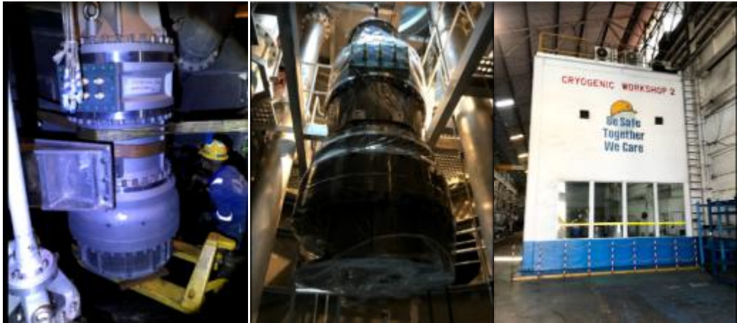
貨泵拆卸/保護/Cleaning Room
